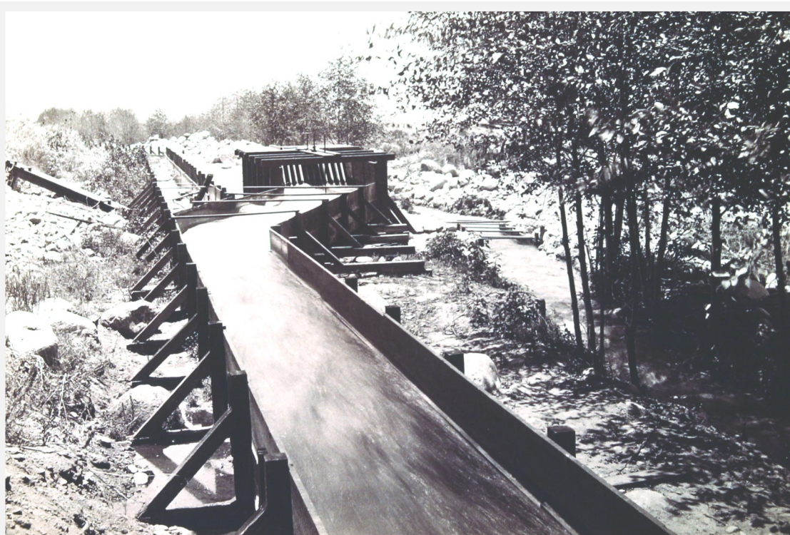
Redwood Flume built by Judson & Brown for the North Fork Ditch.
