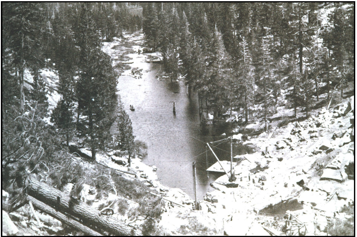
Bear Valley Dam Under Construction in 1883.
