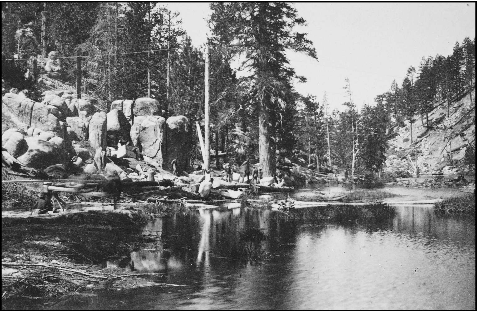
Bear Valley Dam Quarry.
